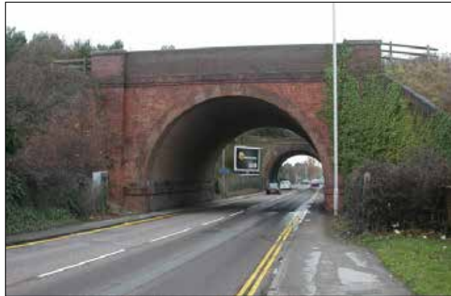
Locally Listed railway bridge on Blandford Road
