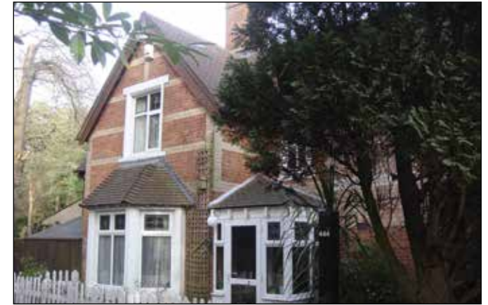
Locally Listed lodge on Blandford Road
