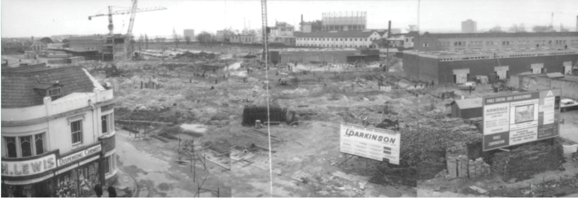
Kingland Road demolition, 1960's
