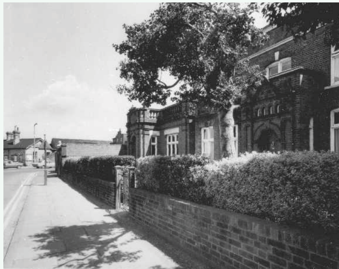
Towngate Street prior to demolition (Poole Museum)
