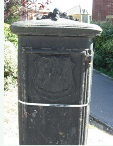
Tram Control Box: North Road
