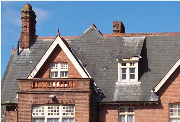
Traditional slate roof
