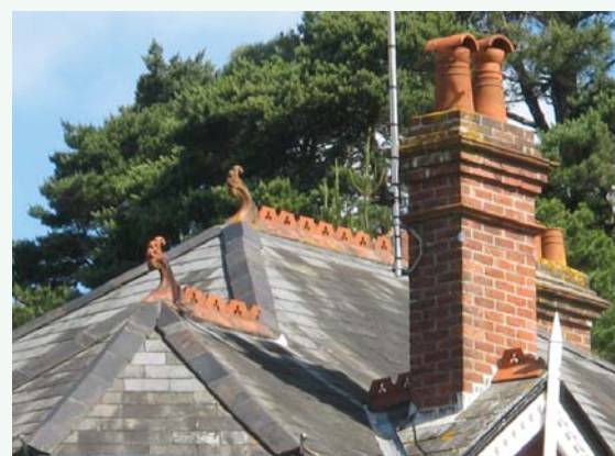
House showing traditional details: Slate roof, finials, chimney and barge board.
