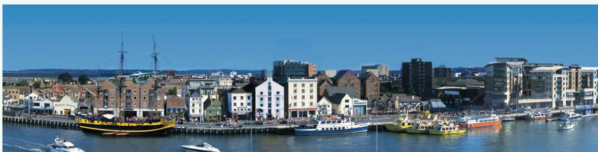
View towards the Quay from the water, showing the varied skyline and prominence of buildings.
