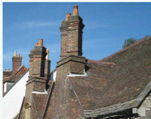
Fine traditional chimney
