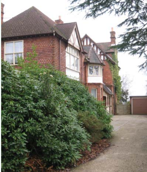
Traditional building with primary façade orientated away from the street
