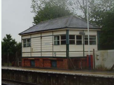
Signal Box, Hamworthy Junction
