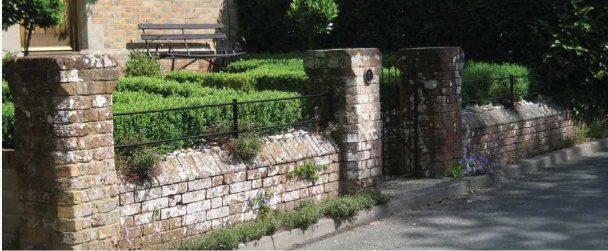
Important front boundary wall
