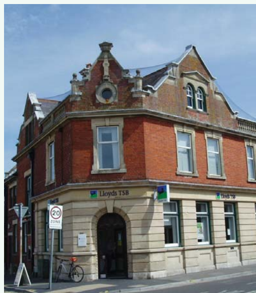
Lloyds Bank Ashley Road A Local Heritage Asset
