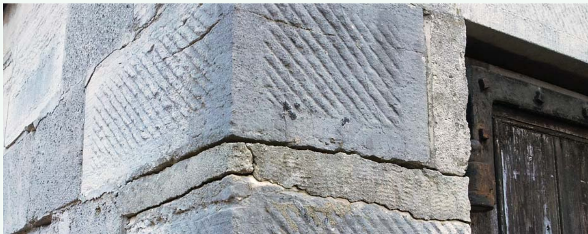
Inappropriate cement mortar, applied on damaged stonework emphasising the joints
