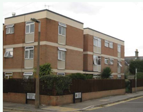
Inappropriate infill development in Heckford Park Conservation Area
