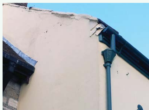
Traditional rainwater goods
