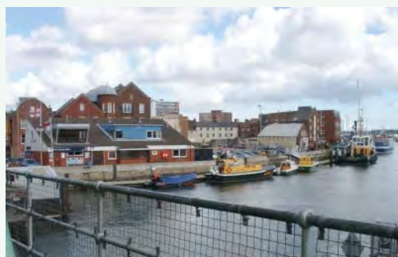
Post-war infill obstructs the views of historic buildings
