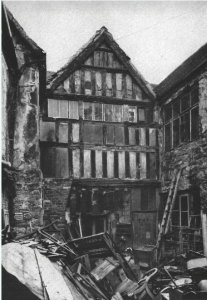
14 High Street, 16th c. timber framing rear elevation
