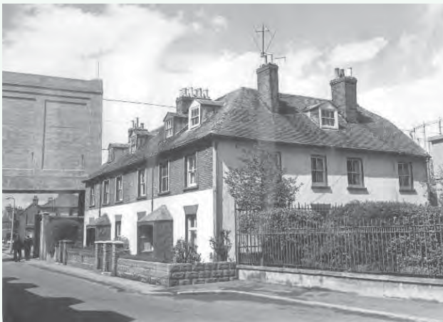
Green Road with the gasworks to the north
