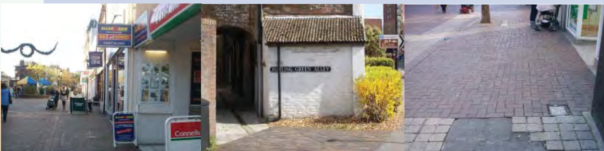
High Street, signage clutter, restored alleyway and poor paving maintenance
