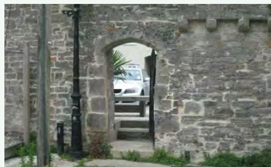
Repaired boundary wall, St. Clements Lane
