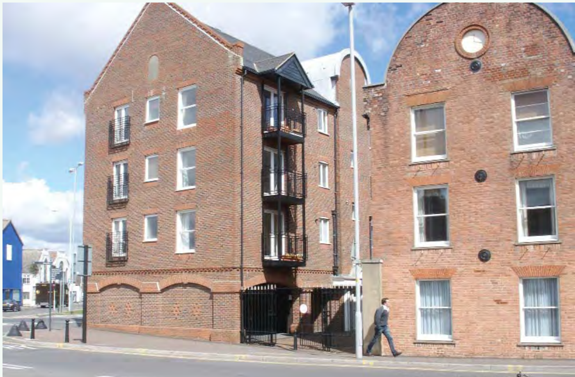
Barbers Gate, good contextual architecture
