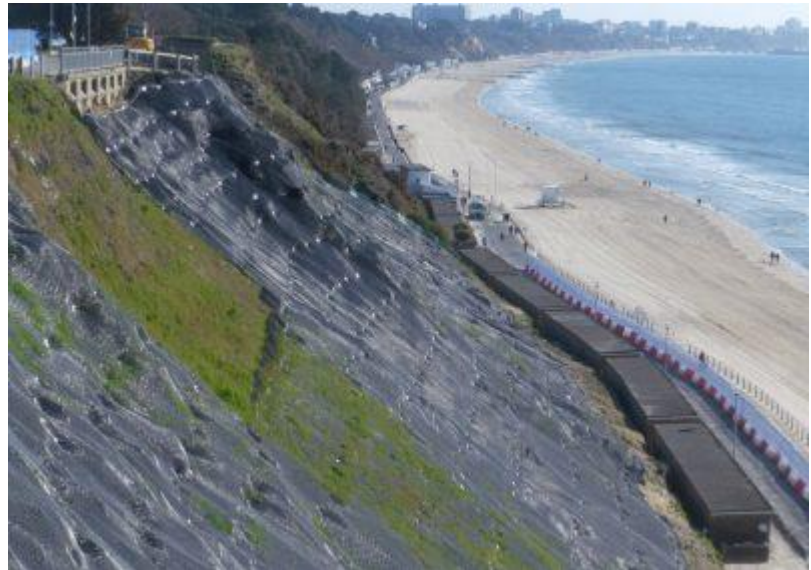
Photo: Cliff erosion protection scheme 2021
