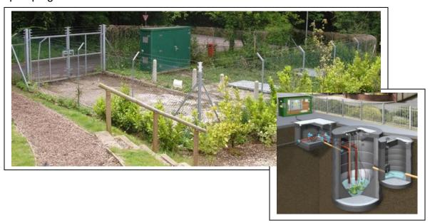
97. Note these images are representative of the type of foul water pumping station and not part of the application. However, they illustrate how the bulk of the operations are underground, with a kiosk above ground. The drainage plans for
