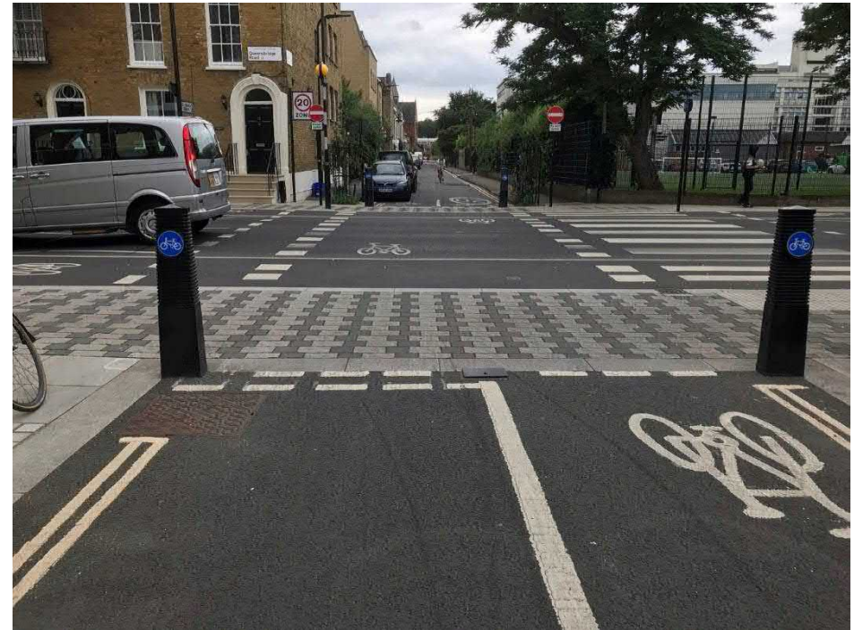
A cycle crossing of a main road in London, between two quiet side streets with restricted entry to motor vehicles. Photo credit: ActivePlanning
