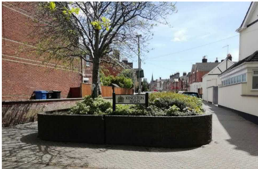
An example of an historic "modal filter" at the end of Kingston Road in Poole. The term modal filter refers to that fact that some modes (cycling and walking) - can filter through whereas others (driving) cannot.
