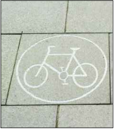
Example of cycle symbol paving unit
